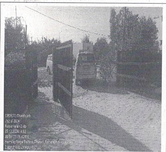
View of Entry Gate of 05 MLD STP, Raipur Kalan-II, Chandigarh
